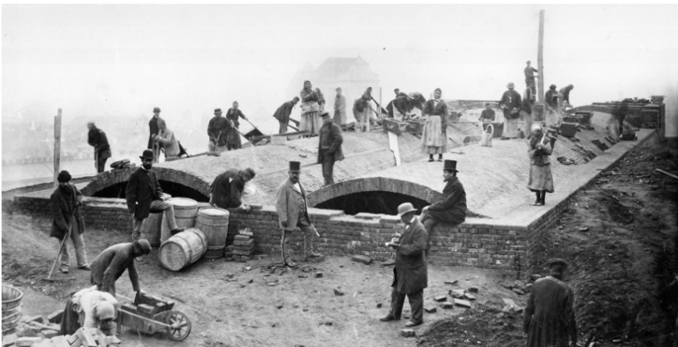
Construction of an older water reservoir (1870 - 71)
