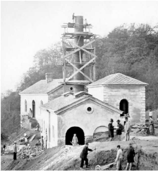
Construction of the pumping station (1870 - 71)
