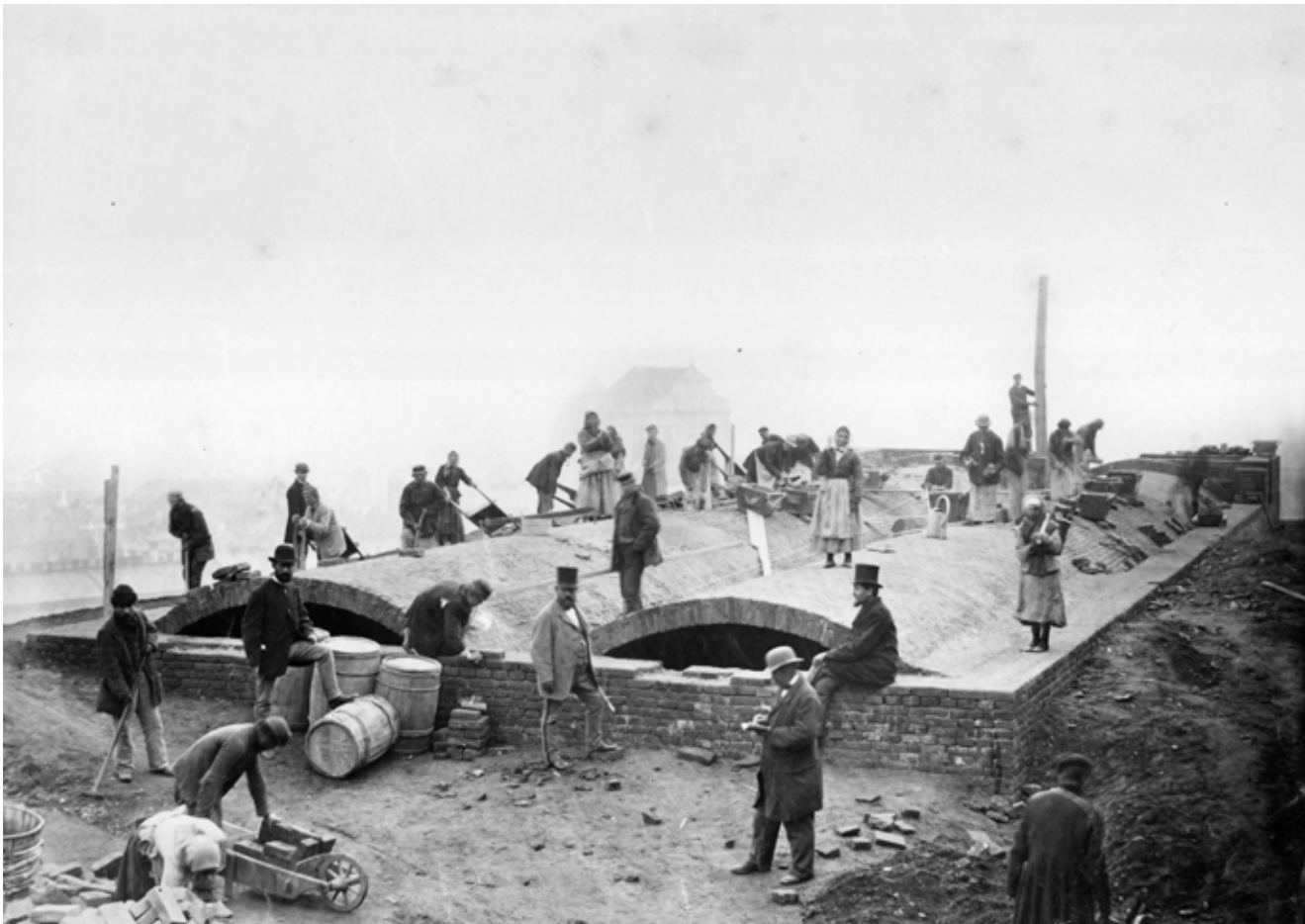
Construction of an older water reservoir (1870 - 71)
