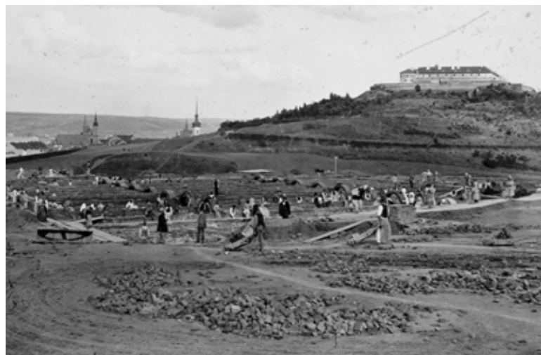
Construction of water reservoir on Žlutý kopec, Špilberk in the background (before 1900)
