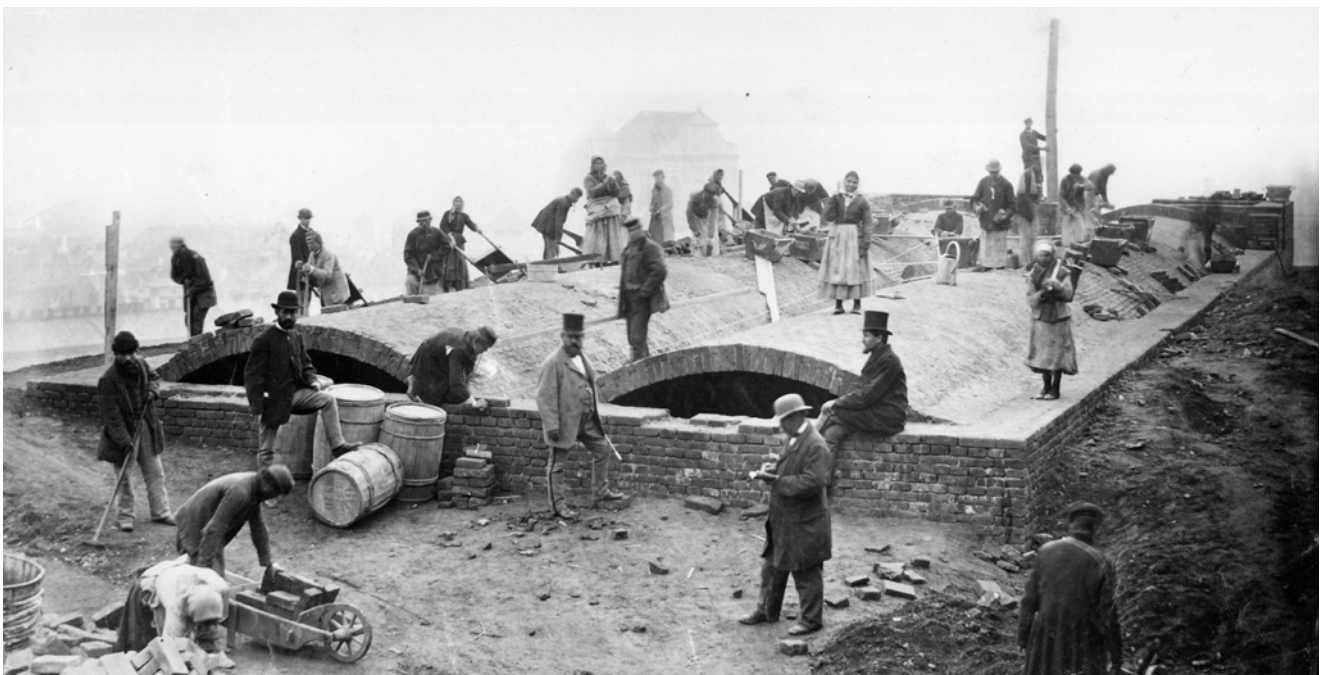
Construction of an older water reservoir (1870 - 71)
