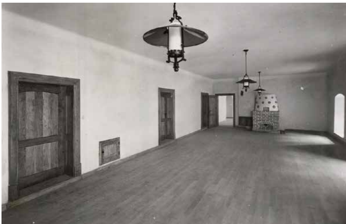
The square tower after the reconstruction for the purposes of the Wehrmacht between 1939 and 1941.
